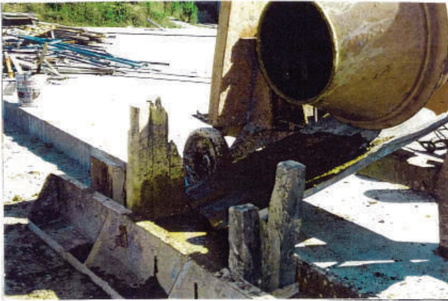
Resim 3.18. Likit Kıvamlı Harcın Kalıba Boşaltılması Picture 3.18. Discharge of Mortar at Liquid Consistency into the Mould
