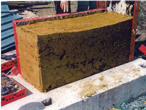
Resim 3.1. Şantiyede Dökülen Numune Blok Picture 3.1. Sample Block Casted in Construction Site
