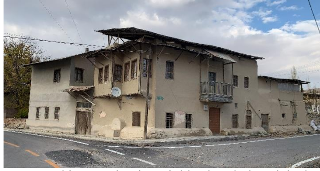
Figure 7. Located on a corner parcel in Hacıderviş Neighborhood, the adobe house has as many spaces and an inner courtyard as a mansion structure. It has double overhang and balcony facing the street. The flat adobe roof was covered with sheet metal in the later period (author's archive, 2022).
