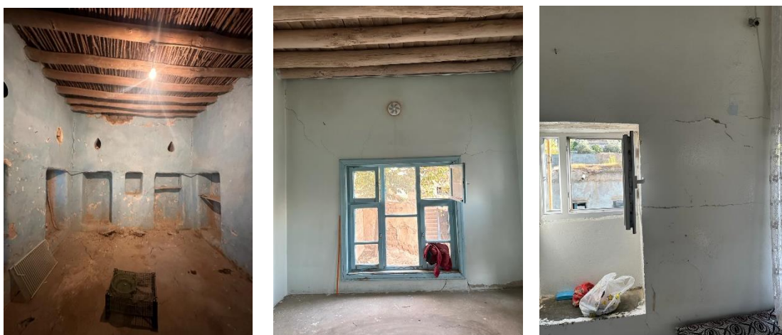
Fig. 6,7,8: Cracks in the walls of adobe buildings in the village due to earthquake (B.B. A. , 2023)
