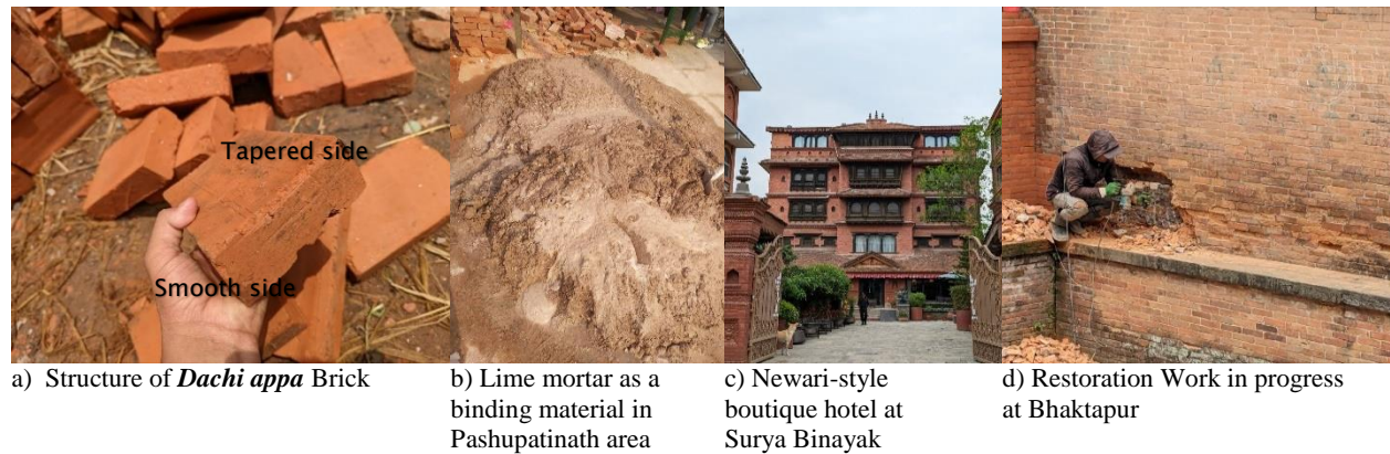
Figure 14: Dachi appa, Lime Mortar, and construction and restoration of structures.
