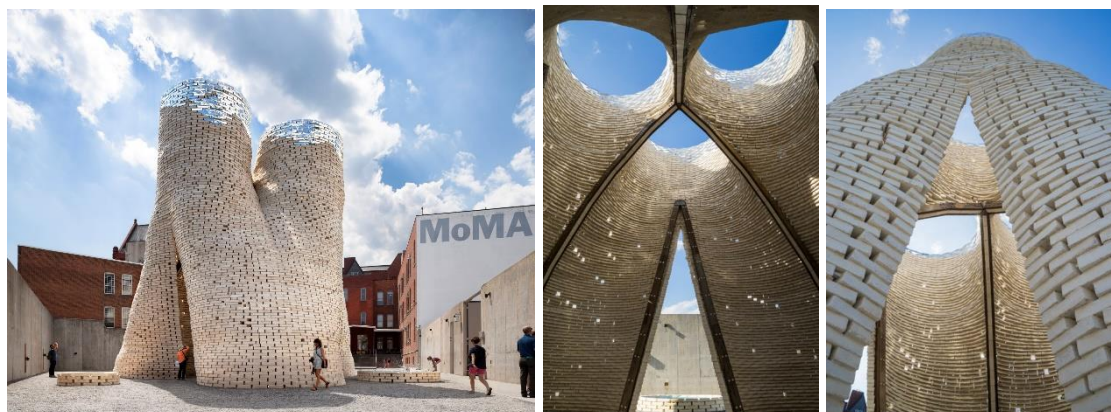
Image 7. The Hy-Fi Tower, compostable mycelium brick structure with zero carbon emissions, 2014 [31] [32]
