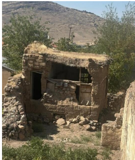
Figure 9: Damage to adobe structure caused by foundation, Zile.
