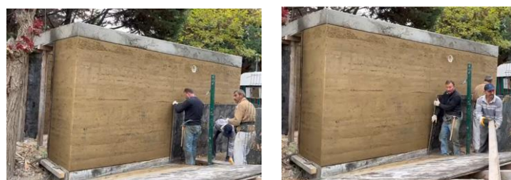
Figure 12. - 13. The Adobe House Whose Molds Were Removed and Made Ready for Roof Construction, Source for Figure 12-13 : Macide Isik Archive
