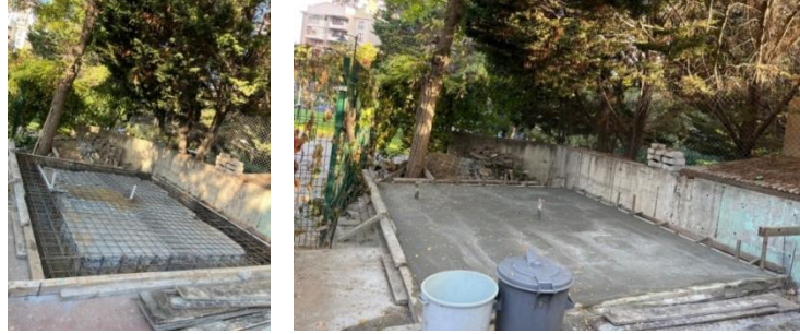
Figure 3. - 4. Reinforced Concrete Foundation of Perma Nature School Adobe House, Source : Macide Isik Archive
