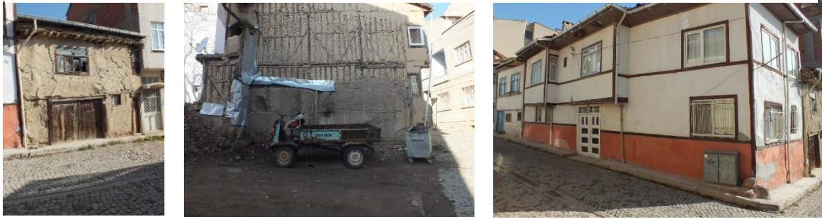
Figure 19 Examples of adobe buildings with wooden construction on Yesildirek Street
