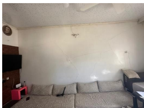
Fig. 9: Out-of-plane damage in Damaged (B.B.A. 2023)
