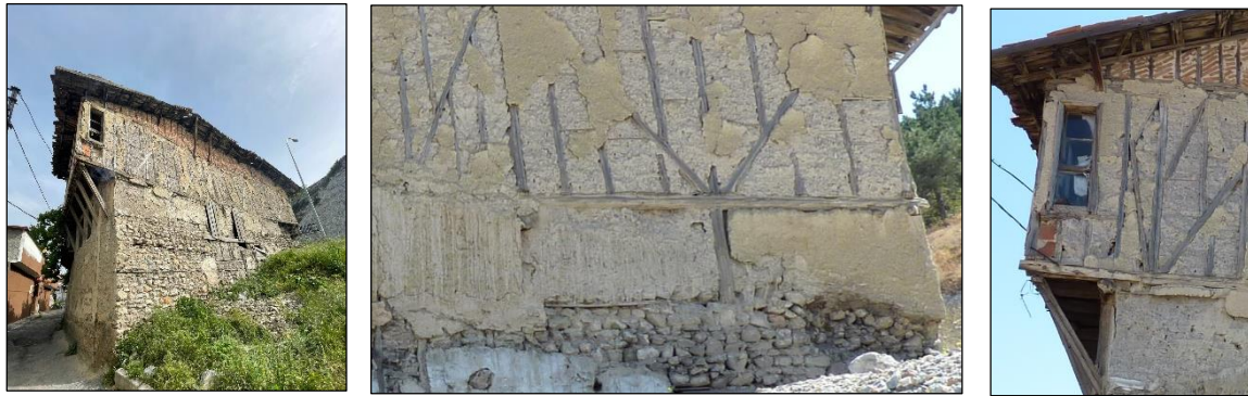
Figure 11. a, b, c. The structural problems and material deteriorations observed on the northeast façade of the building.
