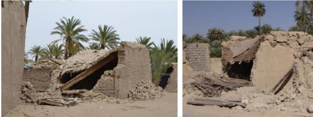
Figure 4. Failure of roof due to out-of-plane wall collapse [9]
