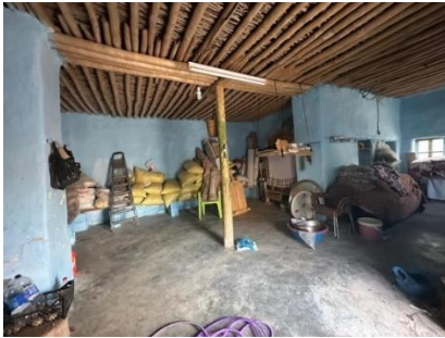
Fig 4: Timber ceiling beams and timber post (B.B.A.2023)
