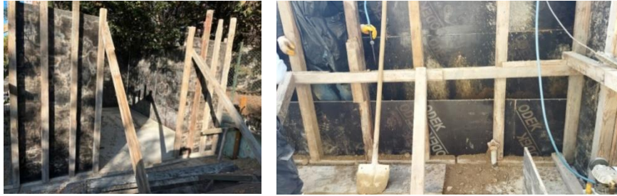
Figure 5. - 6. Formwork Systems Installed for ALKER Building Walls, Source for Figure 5. : Macide Isik Archive, Source for Figure 6. : E. Nurçin Kara Archive
