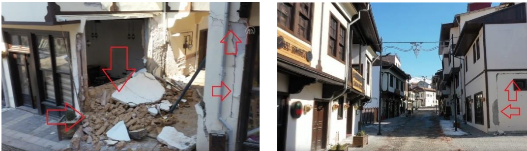
Figure 4. Examples of collapse and cracking of mudbrick walls in Yeşilyurt Mansions (author's archive, 2023).
