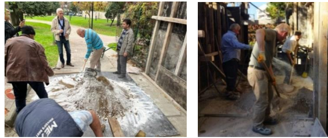
Figure 7. Mixing the Mortar / Figure 8. Wetting the Mortar, Source for Figure 7. : Macide Isik Archive, Source for Figure 8. : E. Nurçin Kara Archive
