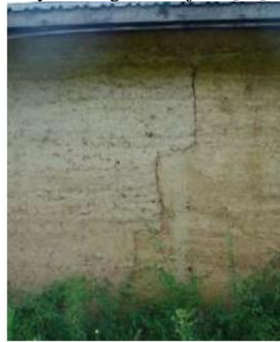
Figure 14: Renovation of the adobe wall by creating stepped work joints [15].
