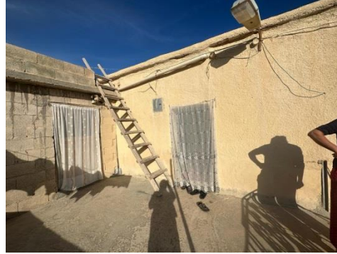
Fig. 3: Adobe House with briquette addition (B.B.A. 1 , (B.B.A., 2023)
