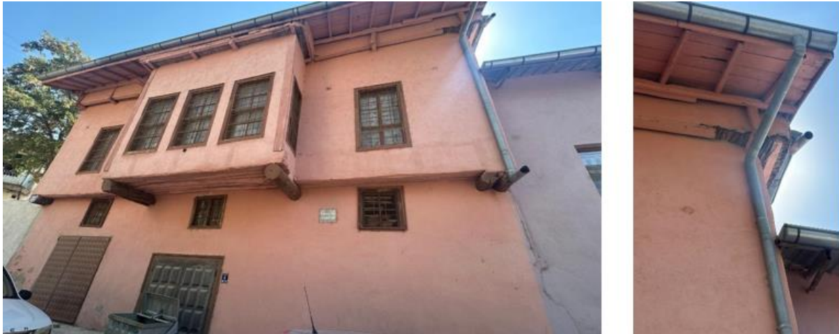
Figure 5: Water damage observed in mudbrick structure, Zile.
