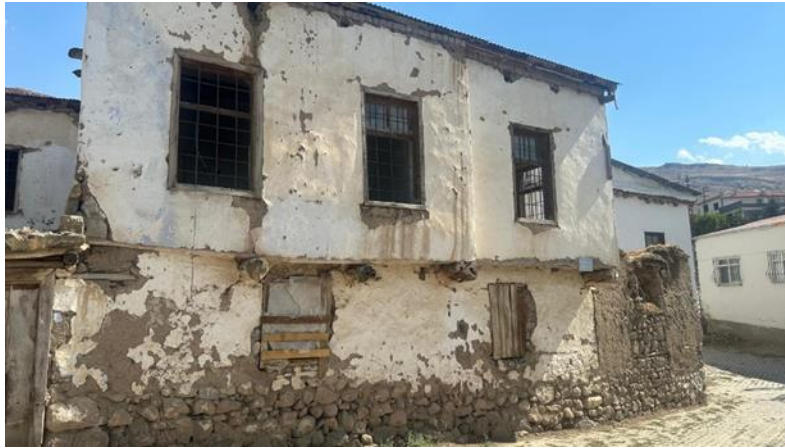
Figure 6: Damage caused by efflorescence on adobe structure, Zile.
