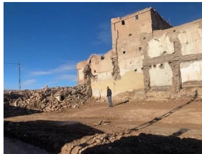
Figure 9. In Darende, the three-storey adobe house that survived the earthquake and the adjacent adobe house, which was completely demolished due to damage and turned into a plot of land, can be seen (URL 4).
