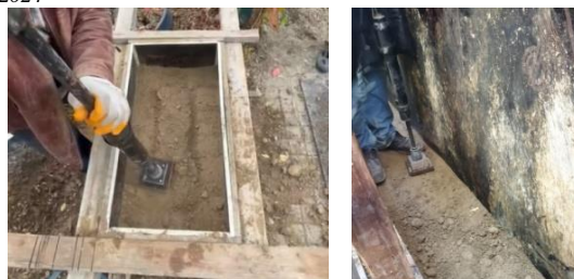
Figure 9. Ramming of the Sample Prepared for Adobe House with Compactor
