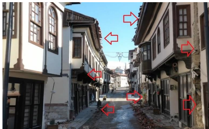
Figure 5. Partial collapse of the roof, eaves and walls of Yeşilyurt Mansions (author's archive, 2023).
