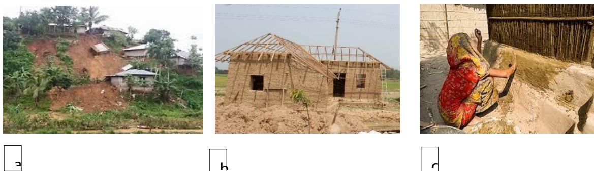
Figure 3: land slide (a), cob construction (b), and repairing wattle-daub house (c)
