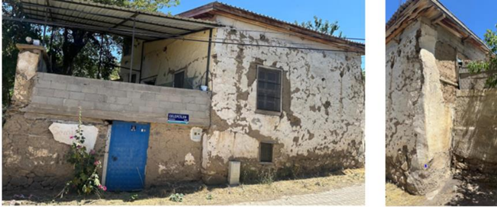
Figure 4: Cracks and damages on mudbrick walls, Zile.
