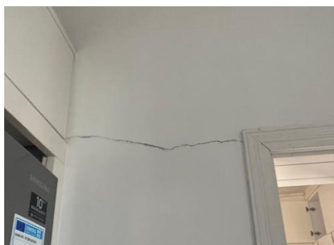
Fig 10: C type Damage in Moderately Damaged (B.B.A. 2023)
