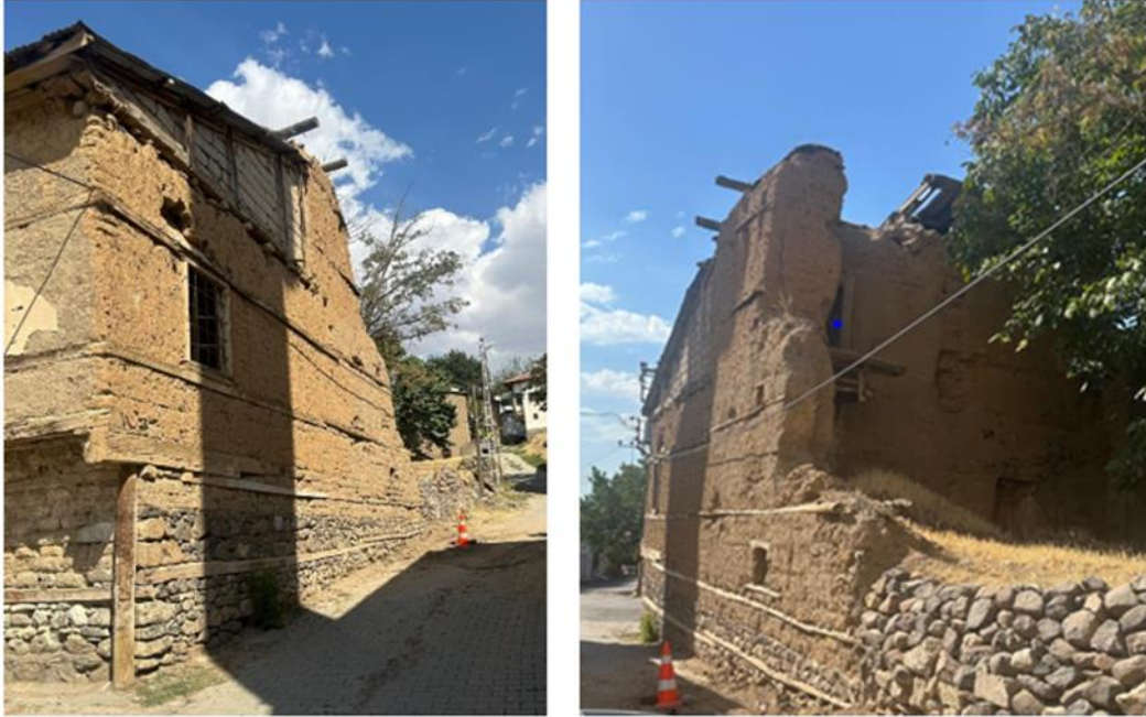
Figure 10: Damage to mudbrick structure due to lack of maintenance, Zile.
