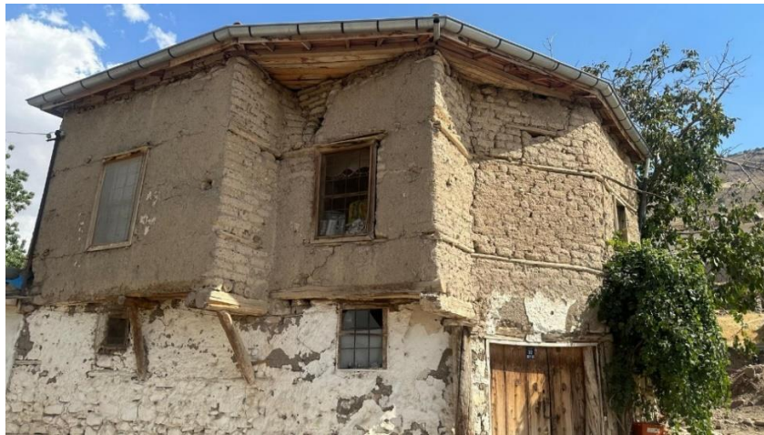
Figure 7: Damage caused by wind and rain erosion on mudbrick building, Zile.
