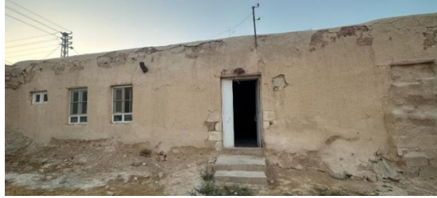
Fig. 11: The building damaged due to ageing as the plaster was not renewed. (Aslan, B.B., 2023)
