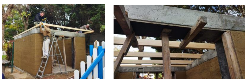
Figure 14 – 15 : Roof Construction after Reinforced Concrete Lintel Construction, Source : E. Nurcin Kara Archive
