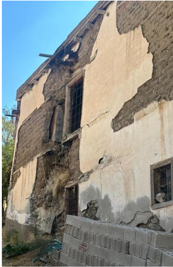
Figure 8: Roof damage to adobe structure, Zile.
