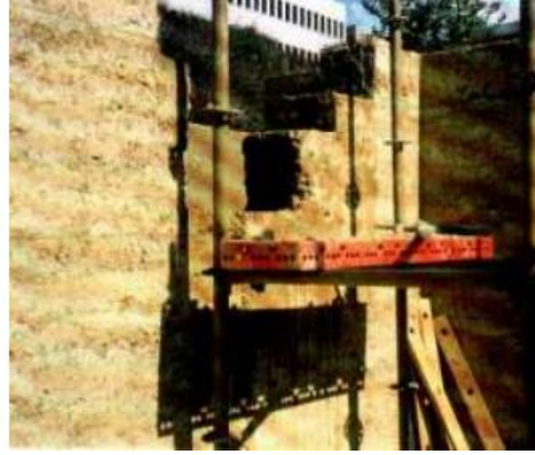
Figure 13: Renovation of the adobe wall by creating a work joint [15].
