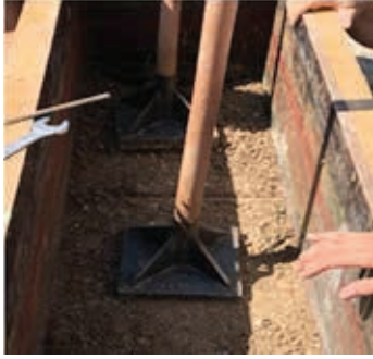
Figure 8. Soil mortar is compressed in a steel mold using a sledgehammer
