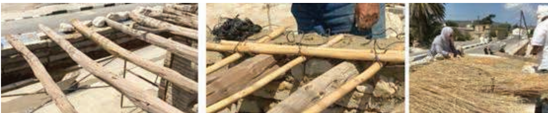
Figure 9. Making the roof construction (G. Benli archive, 2016)
