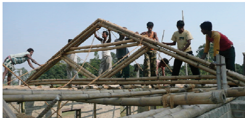
Figure 7. Bamboo truss being put on bamboo post ( source: author )
