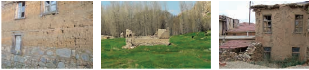
Figure 22,23,24. Examples of deterioration in mudbrick structures
