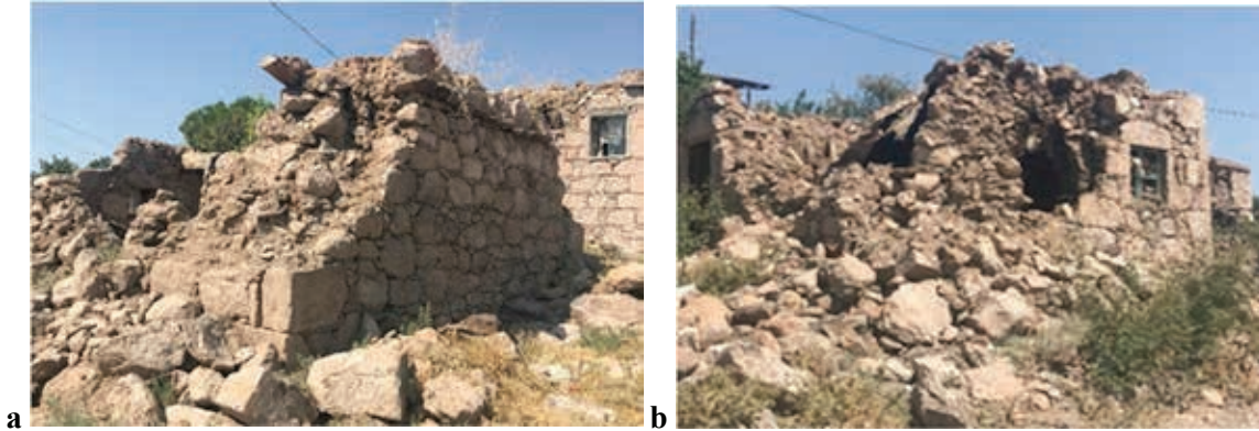
Figure 3. a, b, Using soil as a binder in masonry works.
