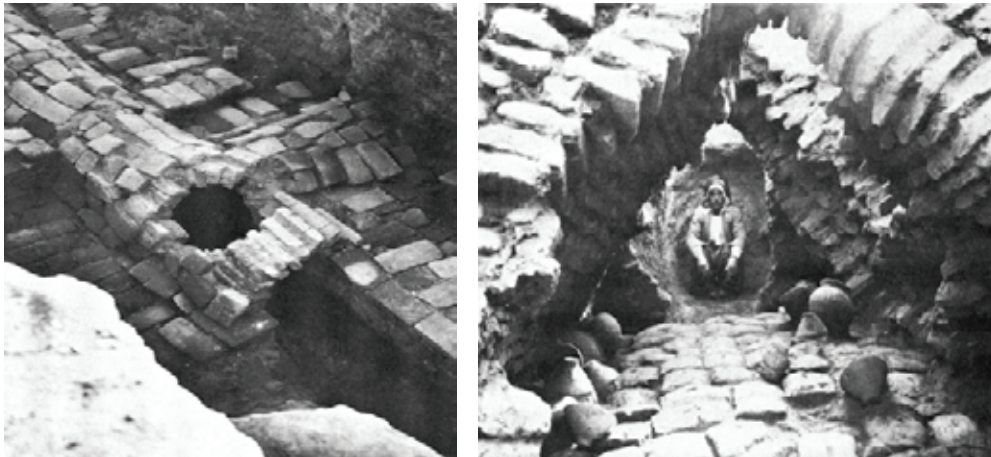
Figure 4. Right: A vaulted sewer of plano-convex bricks Left: A vaulted tomb of baked plano-convex bricks (Lloyd 1967: Plate 40; Delougaz, Hill, Lloyd 1967: Plate 76, 60: B).
