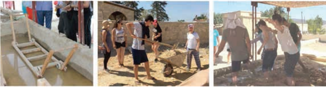
Figure 4. Wooden Adobe Moulds, Mixing Adobe with Straw, Stomping on the Mixture (G. Benli archive, 2016)
