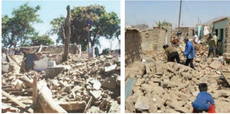
Figure 1. Earthquake destruction of adobe houses Latin America. Left: El Salvador 2001. Right: Peru 2007.
