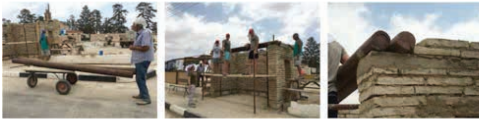
Figure 8. Re-using Lamp Posts as Wooden Beams for the Bus Stop (G. Benli archive, 2016)
