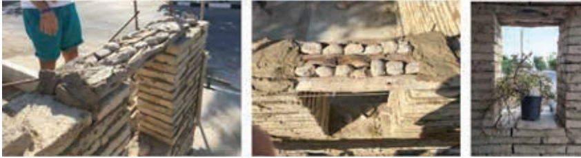
Figure 7. Window Bay and the Production of the Headstall for the Bus Stop (G. Benli archive, 2016)
