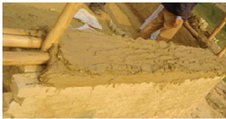
Figure 5. Cob covering bamboo ( source: author )
