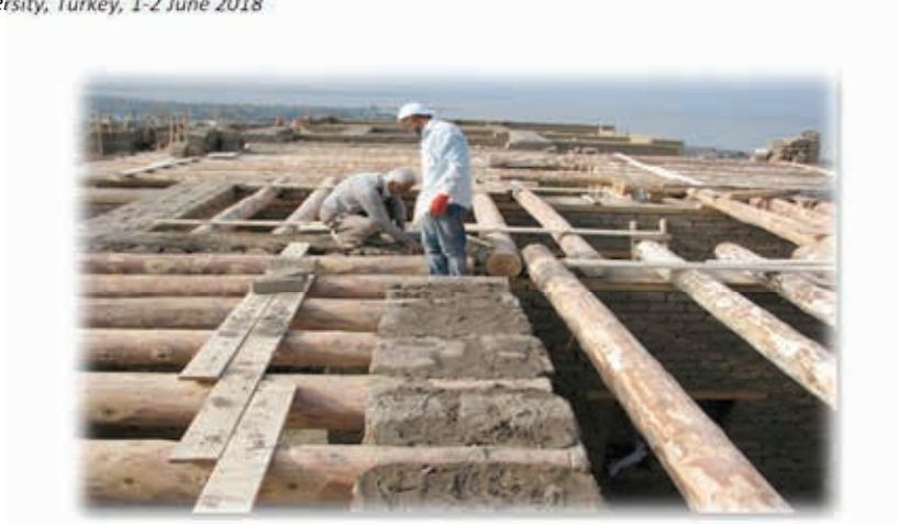
Figure 20. Traditional Van Houses Floor Pavement Construction View (Ş. ÖZTÜRK)
