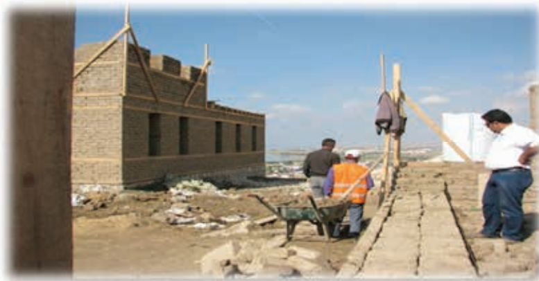
Figure 19. Traditional Van Houses, Mud-brick wall Construction View (Ş. ÖZTÜRK)
