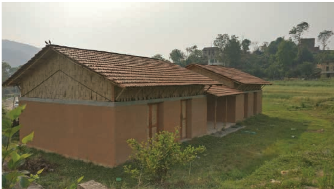
Figure 9. Rammed earth building in Kathmandu University ( source: author )
