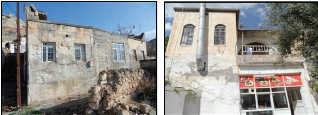
Figure 8. Interventions on facade with unconscious repair works
