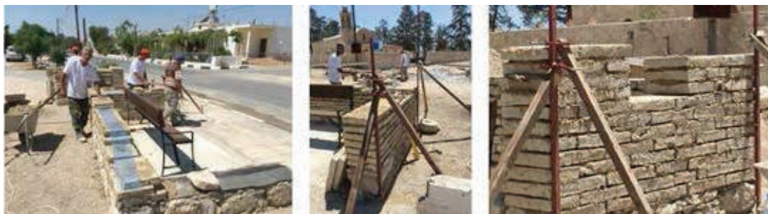
Figure 6. The stages of the laying of the bus stop wall (G. Benli archive, 2016)
