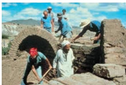
Figure 8. Dar Alsalam Project, New Mexico, USA 1981. The Vaults construction system (url-6).
