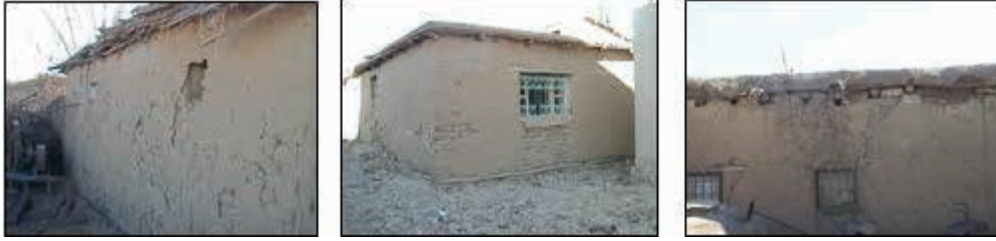
Figure 2. Examples of disruption on the outer surface plaster
